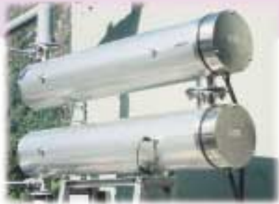
Sewage at Millford Sound is treated using an L Series system
