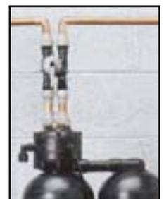
**The Kinetico bypass makes servicing easier**
