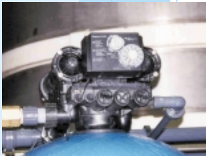
Typical Magnum Valve Installation
